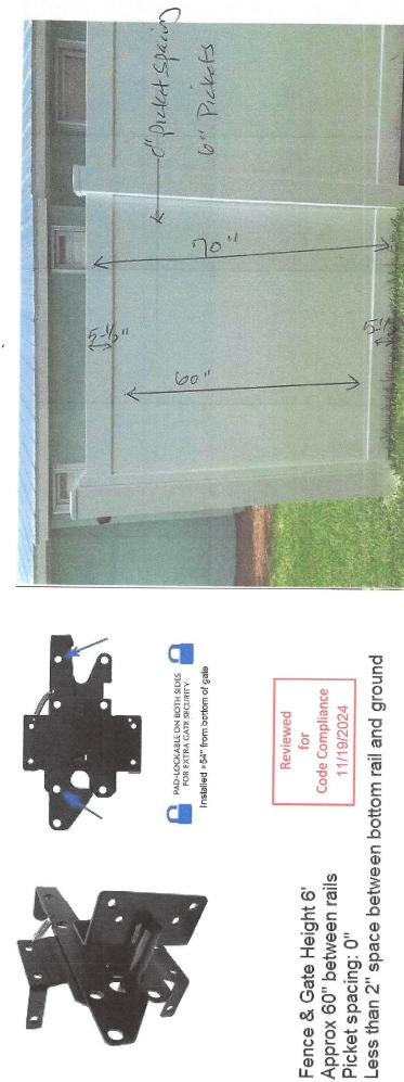
Gate latches installed minimum 54" from bottom of gate Self closing hinges and outward swing on gates
